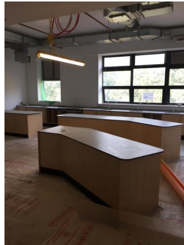
'Fixed Furniture Installed in Science Rooms'
